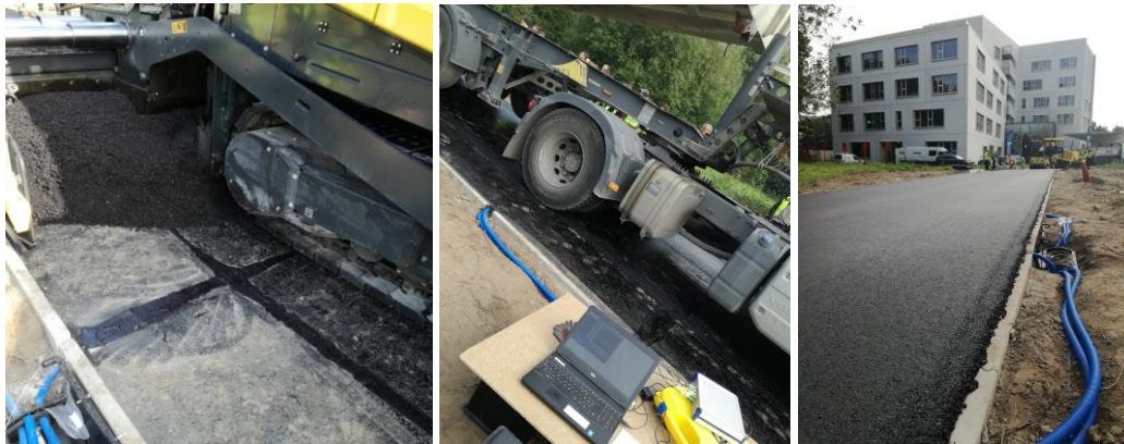
FIGURE 6 Installation of FBGs in two asphalt base layers
